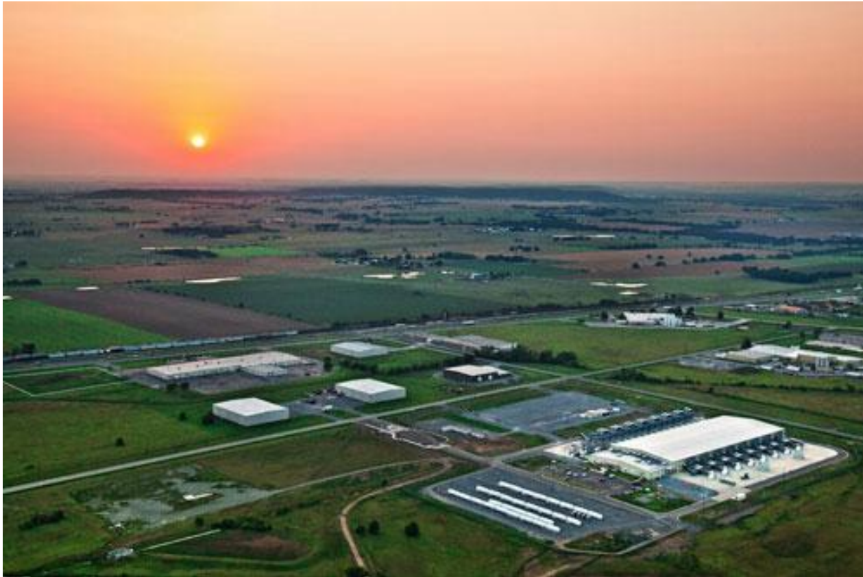
Google's data center in Mayes County, Oklahoma
