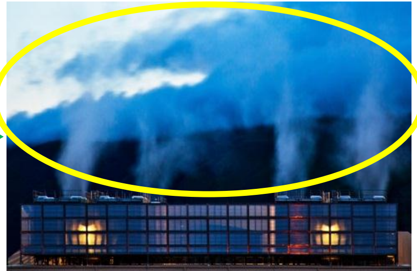
Water evaporation in Google' OR data center
