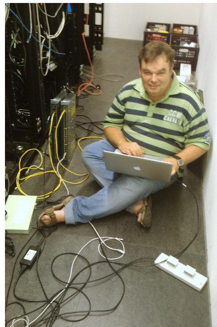
Figure 3: Testing in the data center
